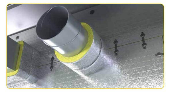
The passage of pipes, electrical cables and ventilation ducts is authorised if they are protected with **U SeaProtect® Roll 46 Alu1** with a thickness of 30 mm to maintain the fire integrity of the B-15 wall extension.
