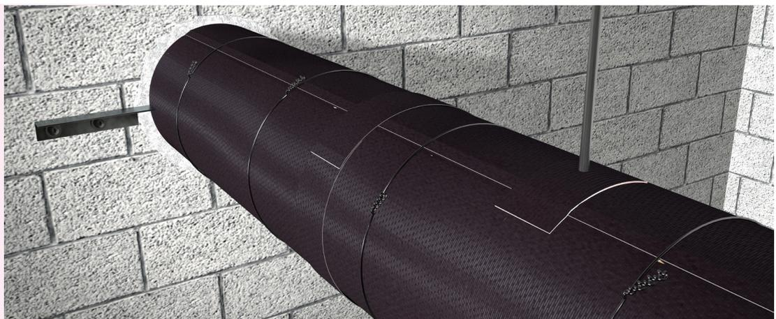
Install the remaining **U PROTECT® VENT SECTIONS** and seal the seams with PROTECT BLACK TAPE. Fix the insulation with 0,7 mm steel binding wire. Max. allowed distance between the binding wires is 250 mm. No need to insulate the hangers.
