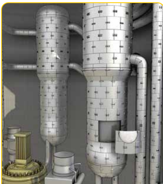
Insulation cassettes on a steam generator
