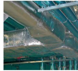
ISOVER solutions for insulation of metal air ducts, installed on the outside of the metal duct.
